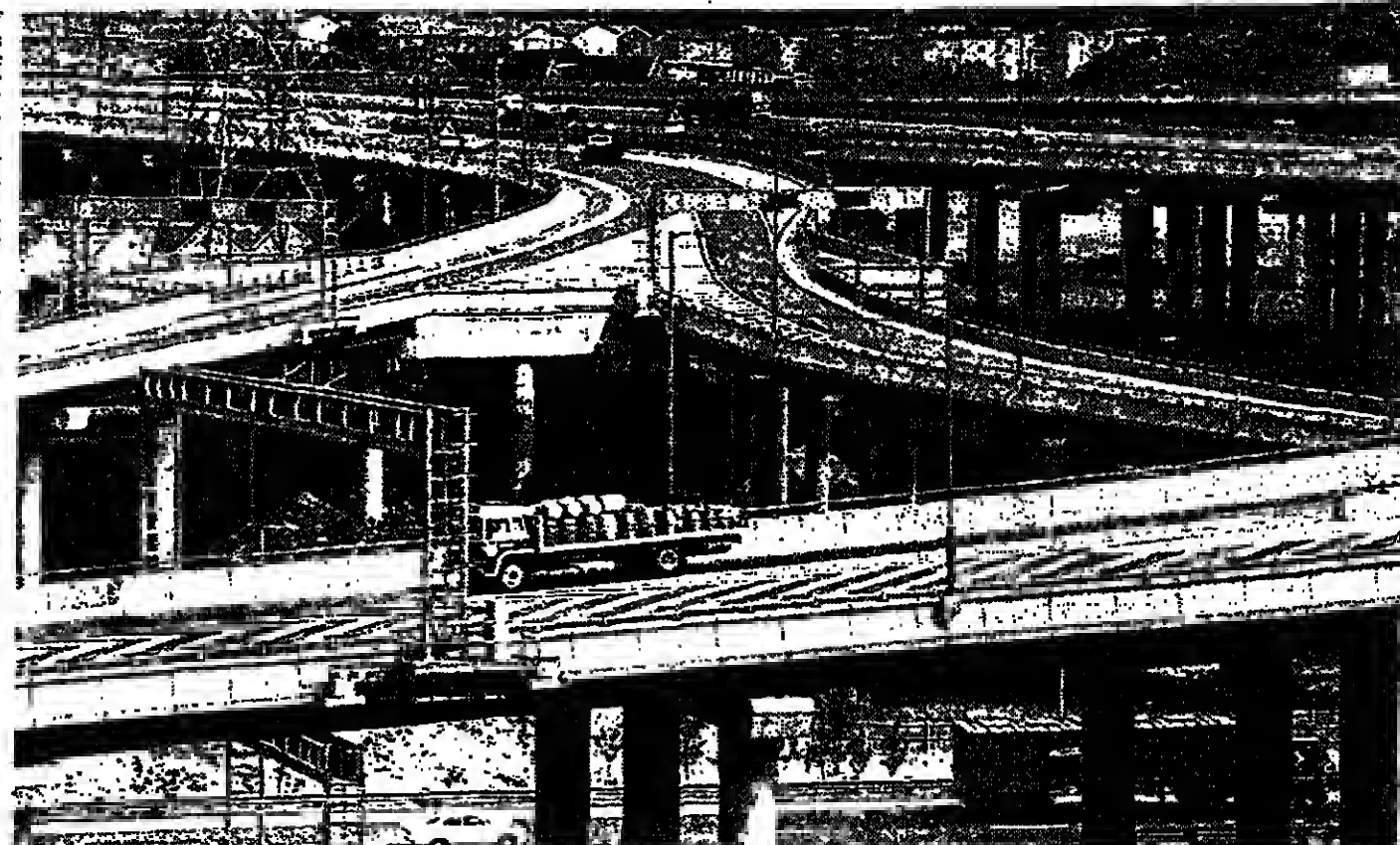
Gravelly Hill motorway interchange. Birmingham's Spaghetti Junction is at the heart of the trunk road network
